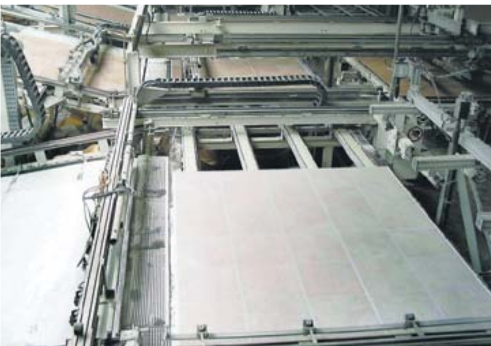
Decorative paper laying station
