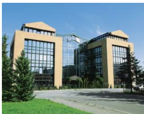
EISENMANN Headquarters, Böblingen
